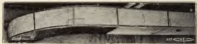
3. Same duct with metal lath soffit. Ready to close in.
